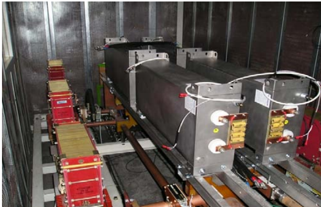
Figure 2 Snubber capacitors installed on a 13kA switch
