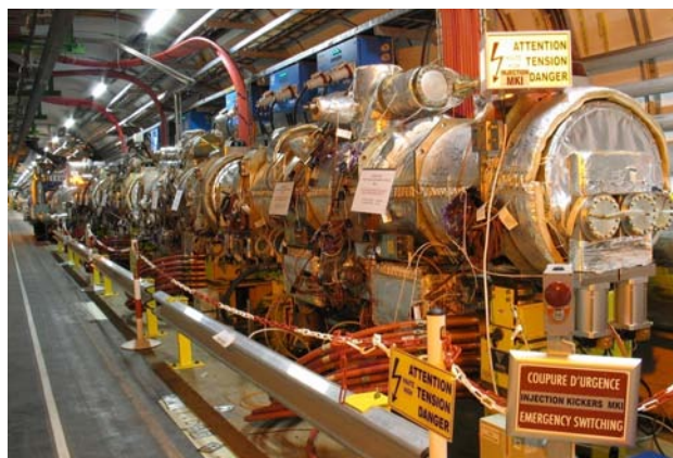
Figure 3: MKI system in LSS8R.
