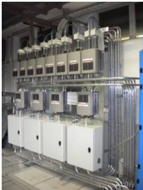
Figure 1: Air sampling smoke detectors with aspiration boxes (in this note referred as non-standard air sampling smoke detectors).
