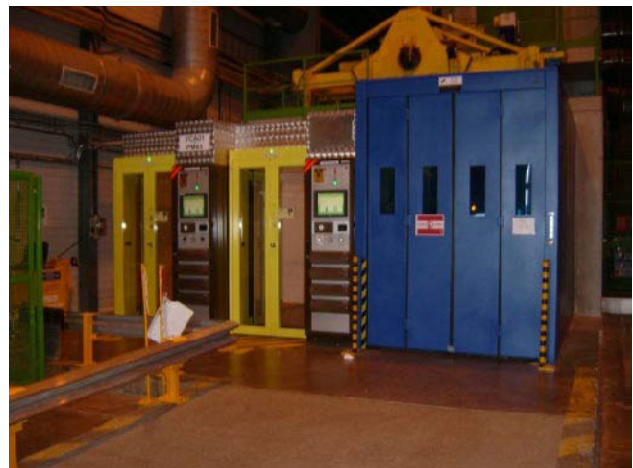
Figure 4: LHC Access System’s access point. Two Personnel Access Devices (PAD) and a Material Access Device (MAD)
