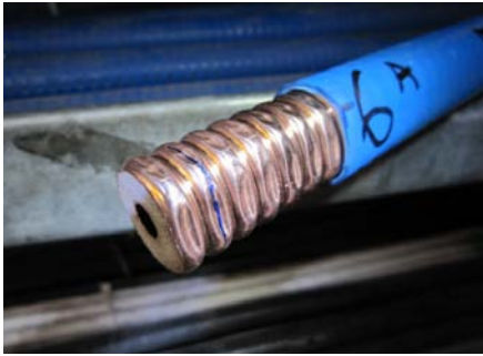
Figure 4: Damaged pick-up cable.
