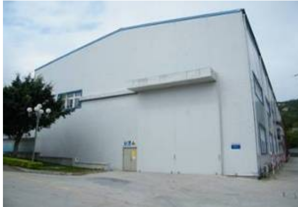
Surface assembly bldg.
