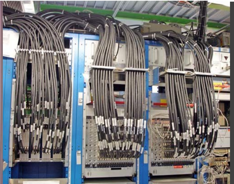
Analogue trigger cables received in electronics cavern
