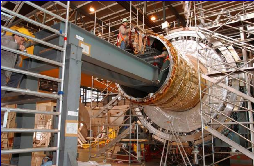
Installation of the solenoid in Feb.2006
