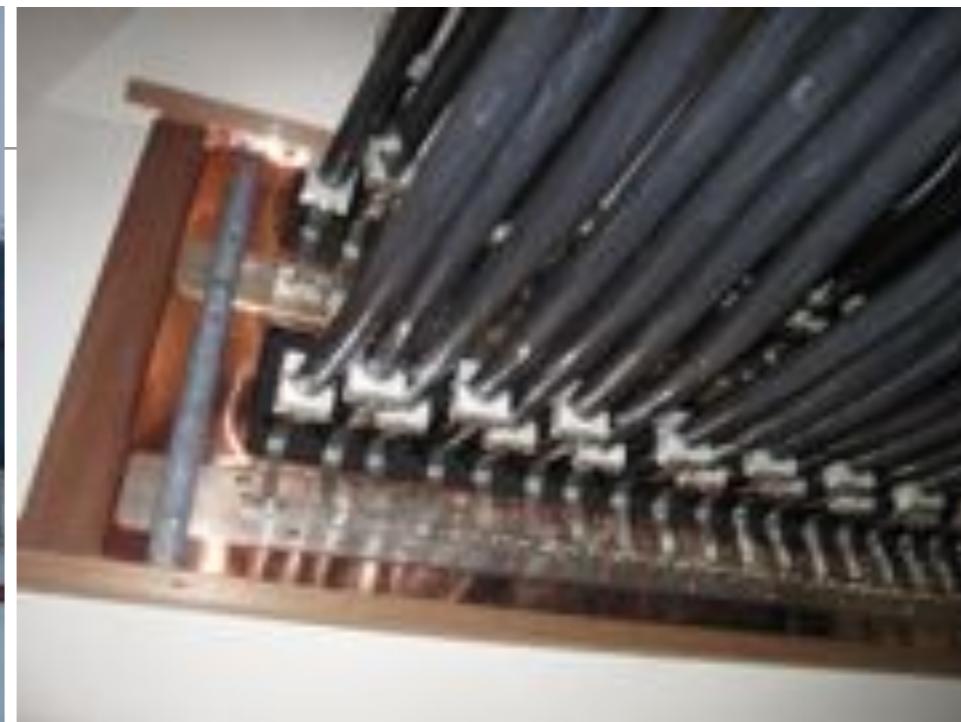
string cable penetrations into ICL
