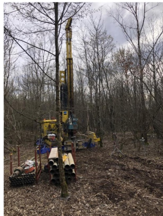
➤ Drilling machine in place
