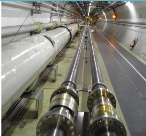
"Twin" sector Beams circulate in different beam pipes
