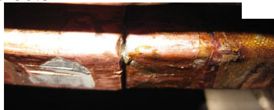
Gap between U-piece and BB stabiliser
