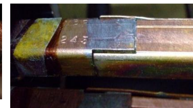
Gap between U-piece and busbar tongue
