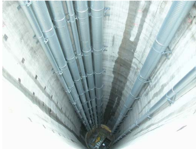
Cooling and Ventilation
