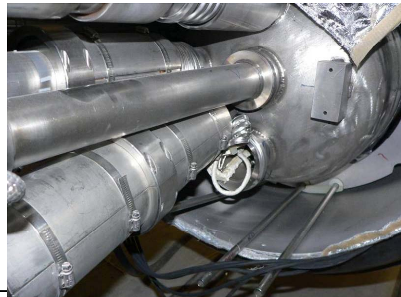
Damaged connections after pressure test failure
