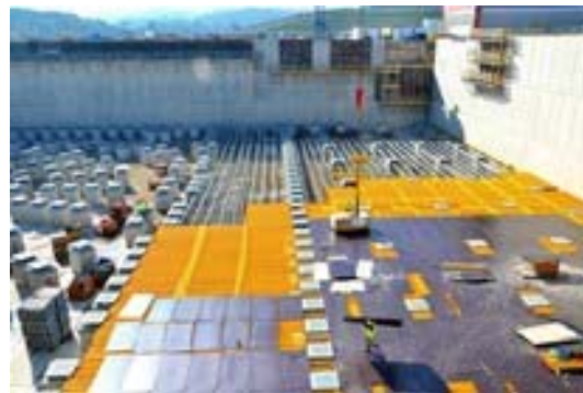
Tokamak Building Pit and Seismic Isolators (17 m deep; 120 x 90 m) B2 slab started
