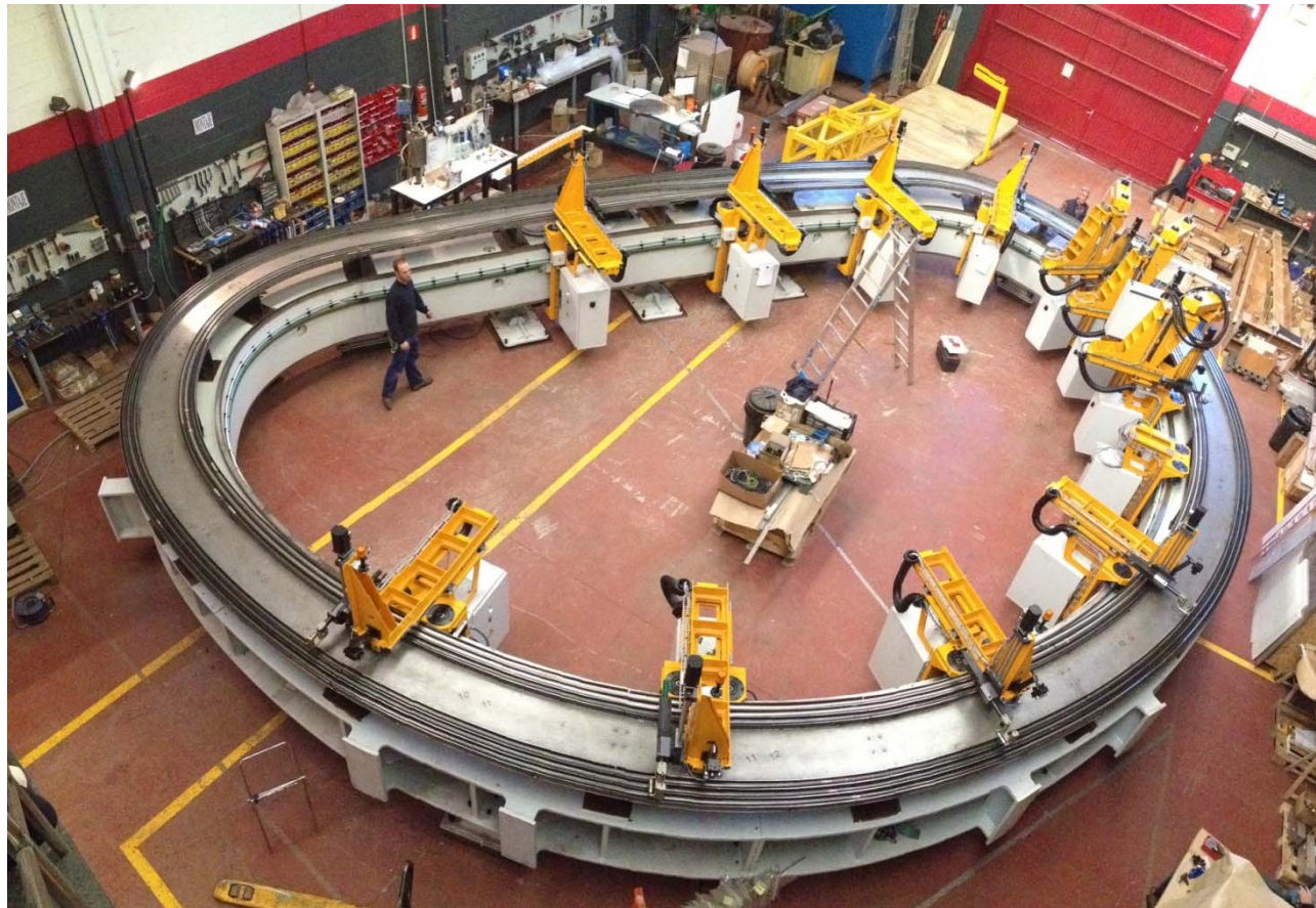
Wrapping tooling for turn insulation of double pancake during assembly at Elytt (Bilbao, Spain)
