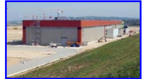
PF Coil Winding Building (17 m high; 252 x 45 m)
