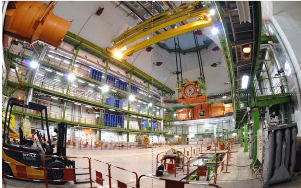
lowering of the HF (very forward HCAL), 2. Nov. 2006
