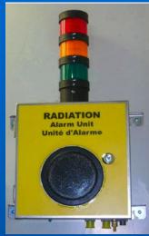
« Gate Monitors » are installed at the experimental cavern exits, with constant link to ACR, to monitor the level of radiation of the equipment leaving the cavern
