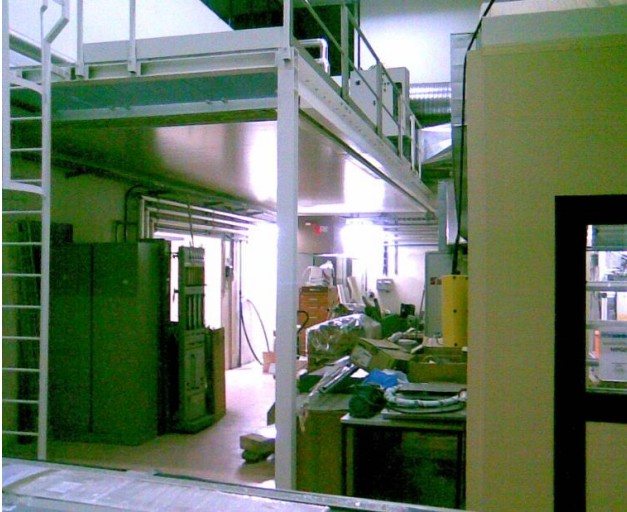
Platform for Air Conditioning Installed
