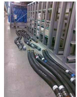
Water Cooled cables removal
