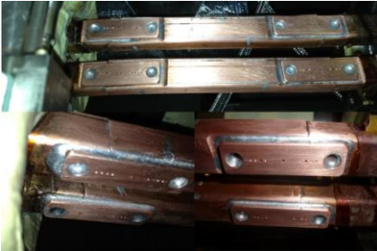
1 st shunt resolder 26/04/13
