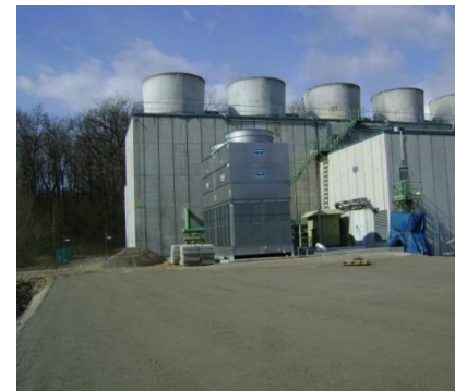
New cooling tower @ P6
