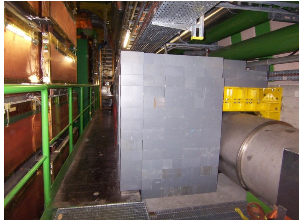
New shielding behind M5
