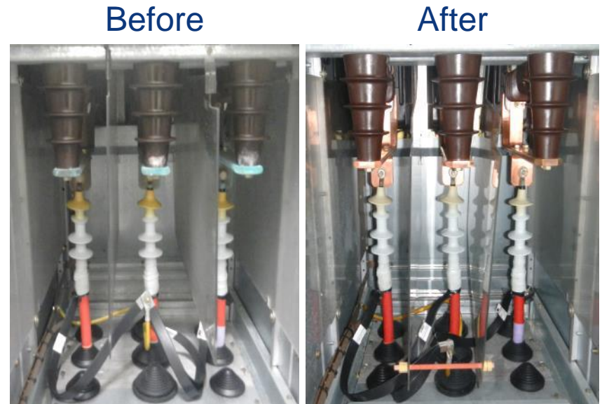
18 kV & 3.3 kV circuit breakers
