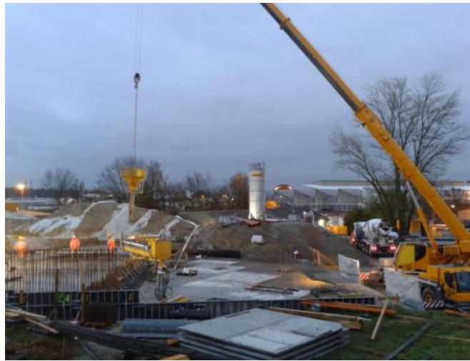
Septum 16 shielding - formworks
