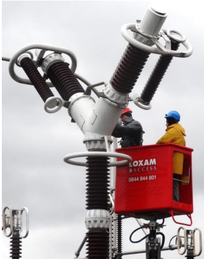
400 kV & 66 kV circuit breakers
