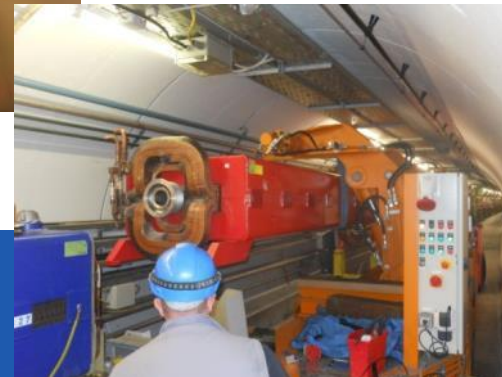
SPS magnet exchange
