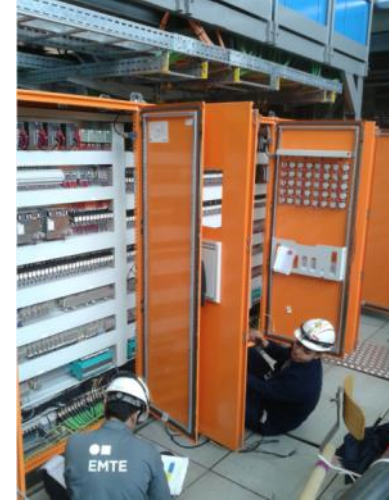
CV cabling works
