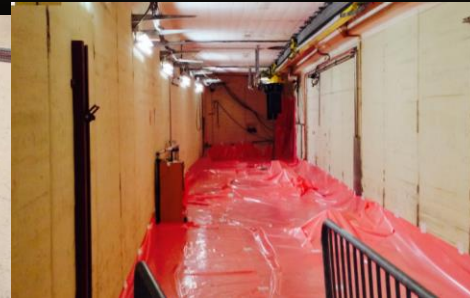
Preparation of the 375-T8 tunnel in order to contain surfacic contamination in view of target removal and movement
