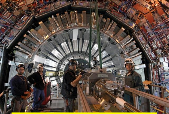
Extraction of CMS beam pipe
