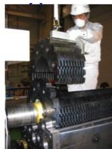
Top Yoke Installation
