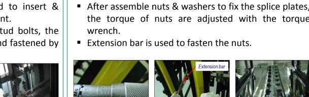
Assembly procedure of VVTS field joint
