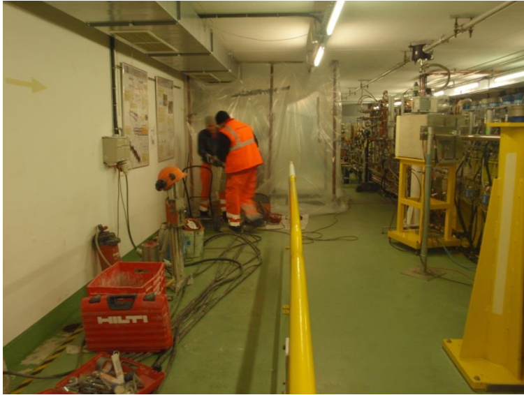
January 2014: Trench cut on the floor and holes drillings through the external wall (2.8 m)
