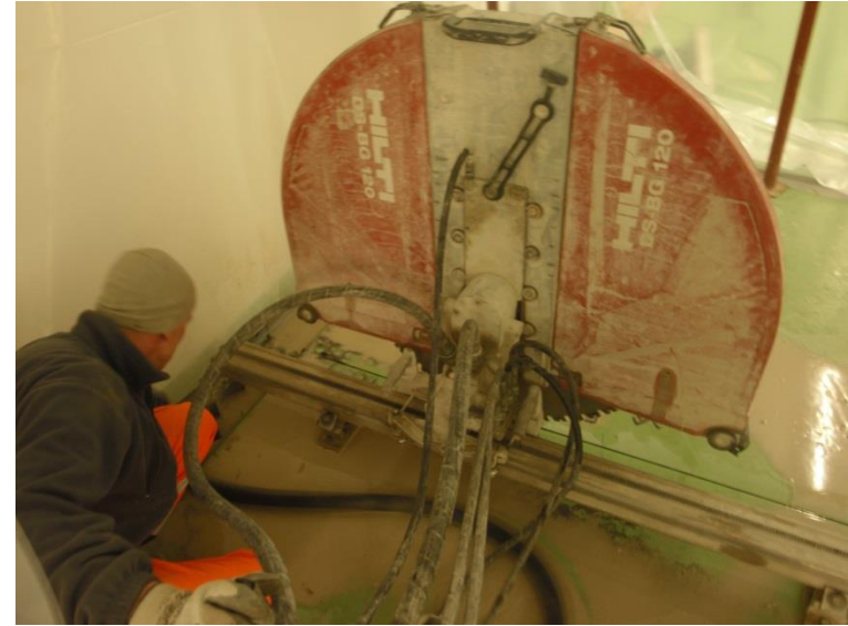
January 2014: Trench cut on the floor and holes drillings through the external wall (2.8 m)
