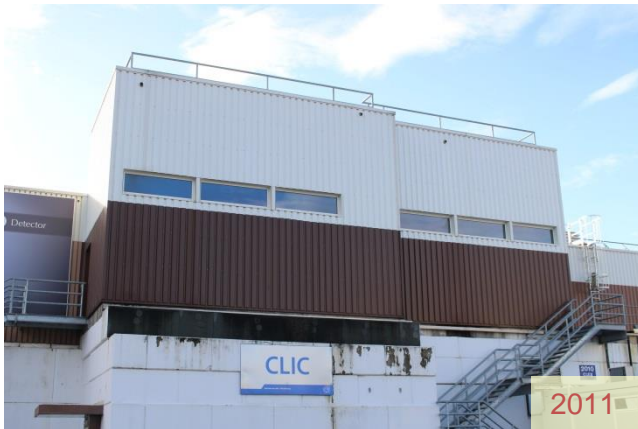
Klystron servicing hall
