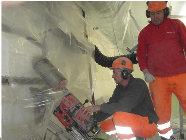
January 2014: Trench cut on the floor and holes drillings through the external wall (2.8 m)
