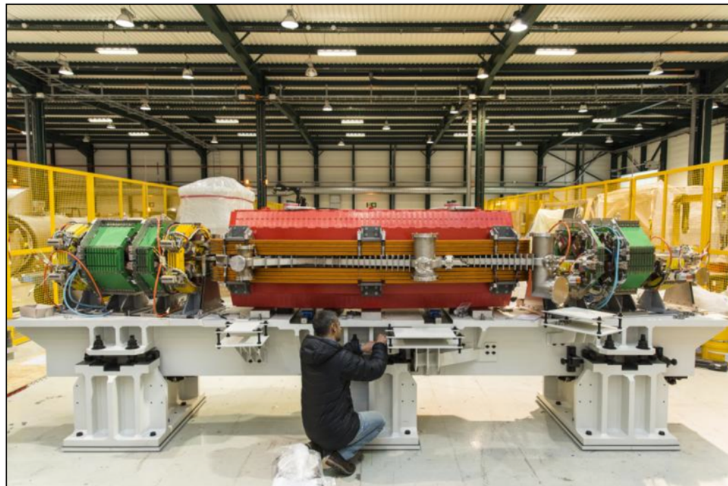
An engineer tests the installation of a vacuum chamber for SESAME, at CERN's magnet-testing facility SM18 (Image: Maximilien Brice/CERN)
