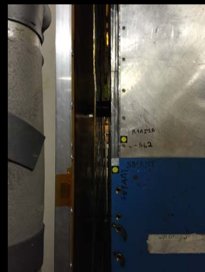
HCC detector in place next to LHCb's RICH & TT1 detectors
