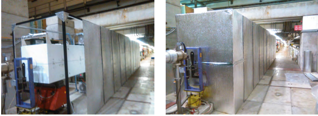
Fig. 35: CEDAR tent structure constructed in 2014.
