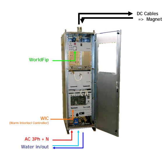
LHC600A-40V Racks were modified to support up to 3 cables / polarity during UJ76 Installation.
