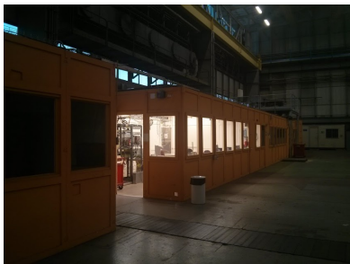
T9 control room
