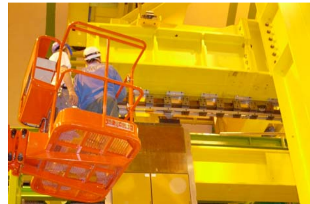
SPD and PS being installed
