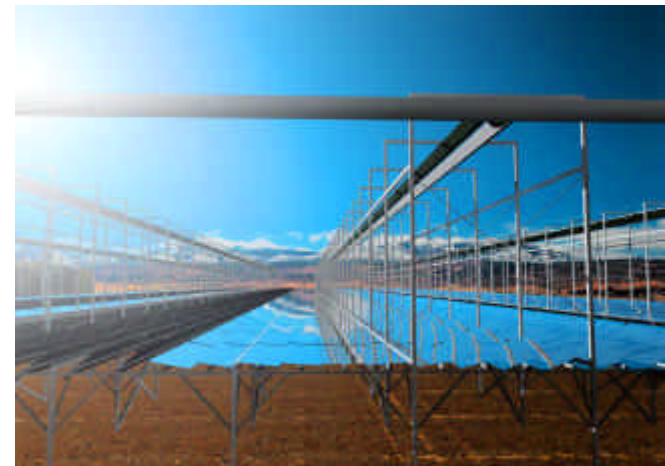
Linear Fresnel reflector
