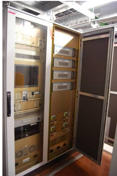
Picture: Temperature controlled EMC Racks housing 6 electronic chassis for the 13kA High Precision DCCTs for the LHC main power converters
