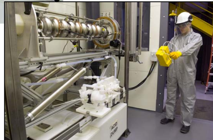
New electro-polishing facility at Argonne
