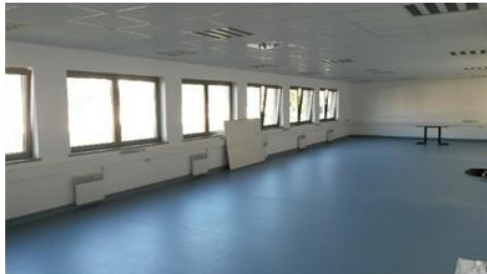
New ISOLDE Control room in B508
