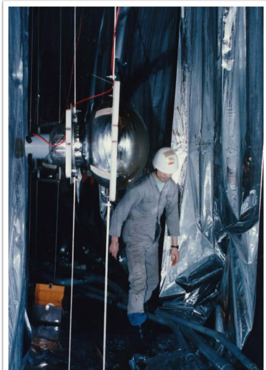
Construction of the side outer detector (between the steel tank and the rock)
