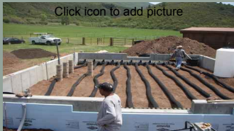
Climate battery installation
