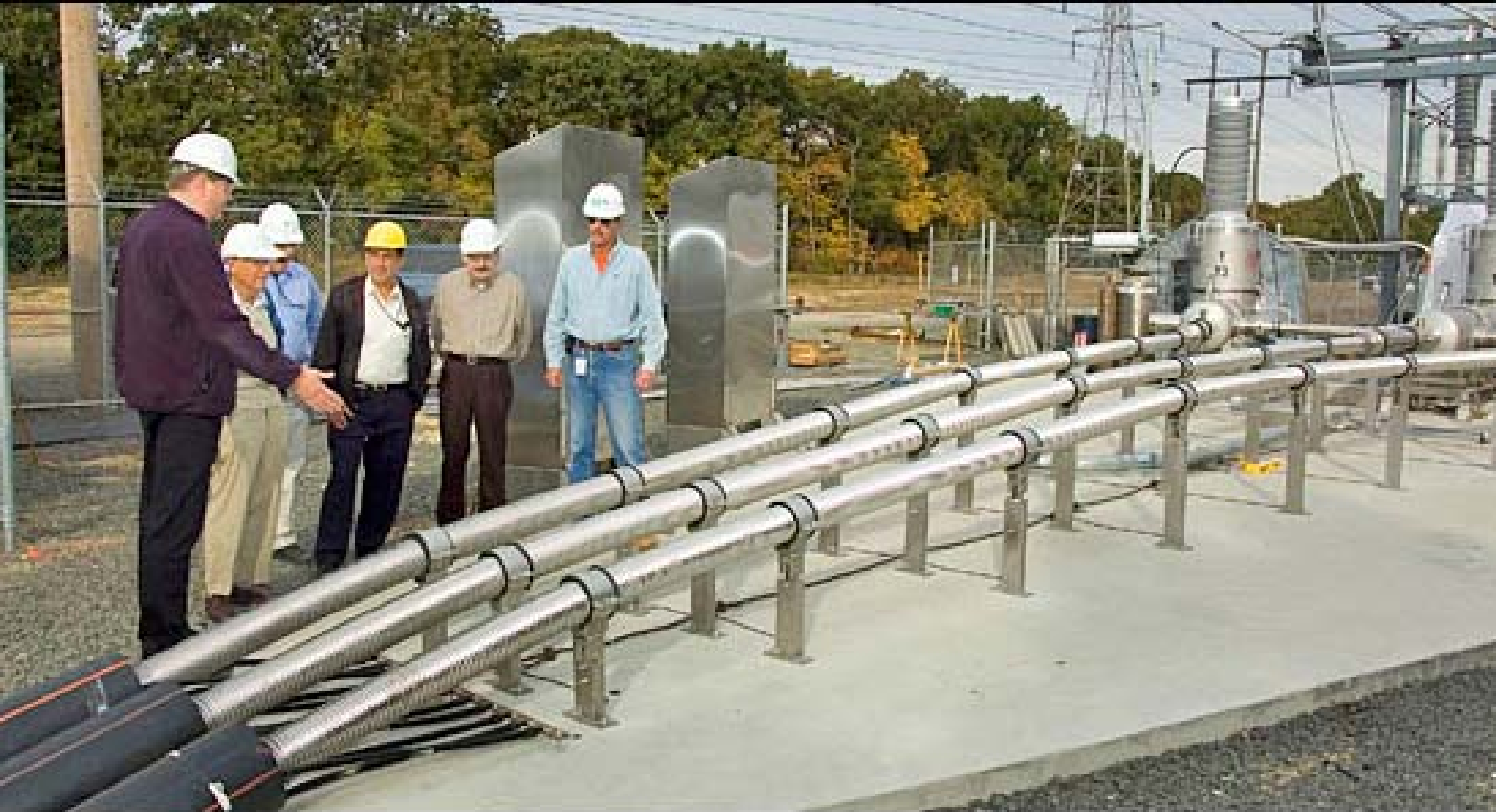
the pipes containing the HTS cables, capable of carrying 574 megawatts of power in a four-foot right of way.
