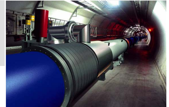
Illustration of LHC dipole in tunnel
