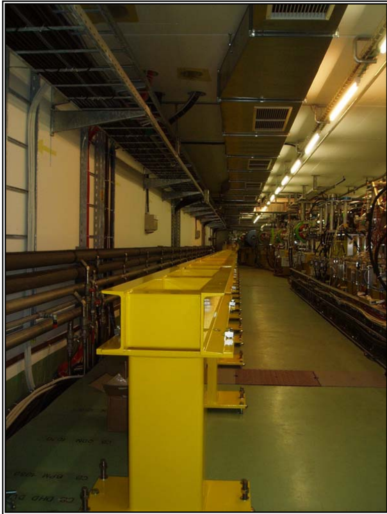
Beam line girders
