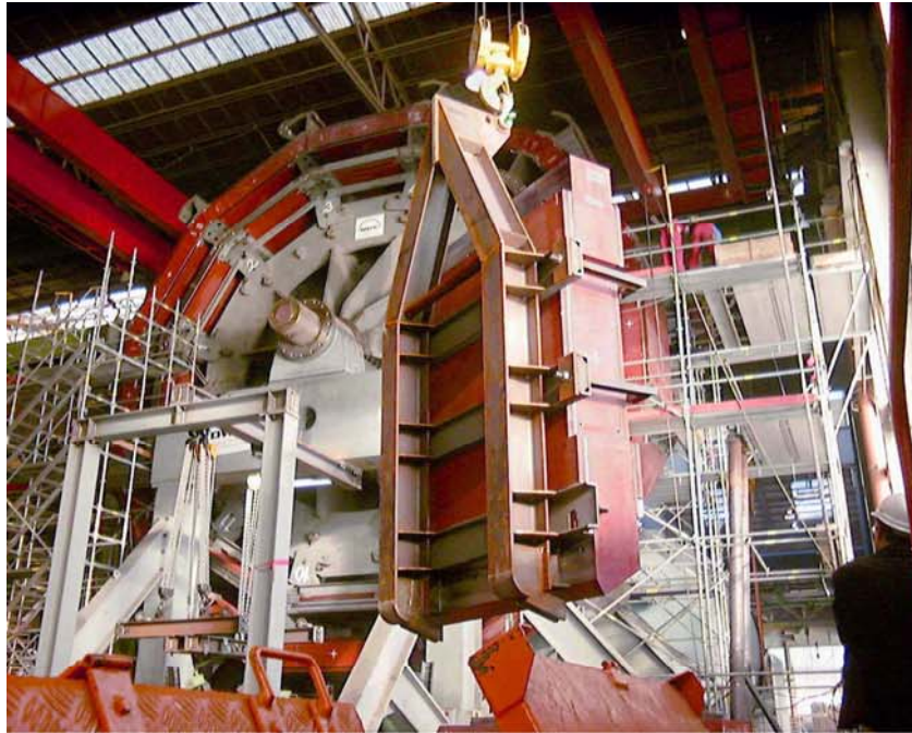
Pre-assembly at Deggendorf (1999)
