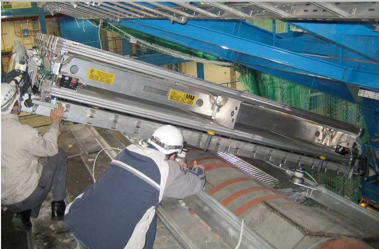
Installation of a Barrel Muon Station
