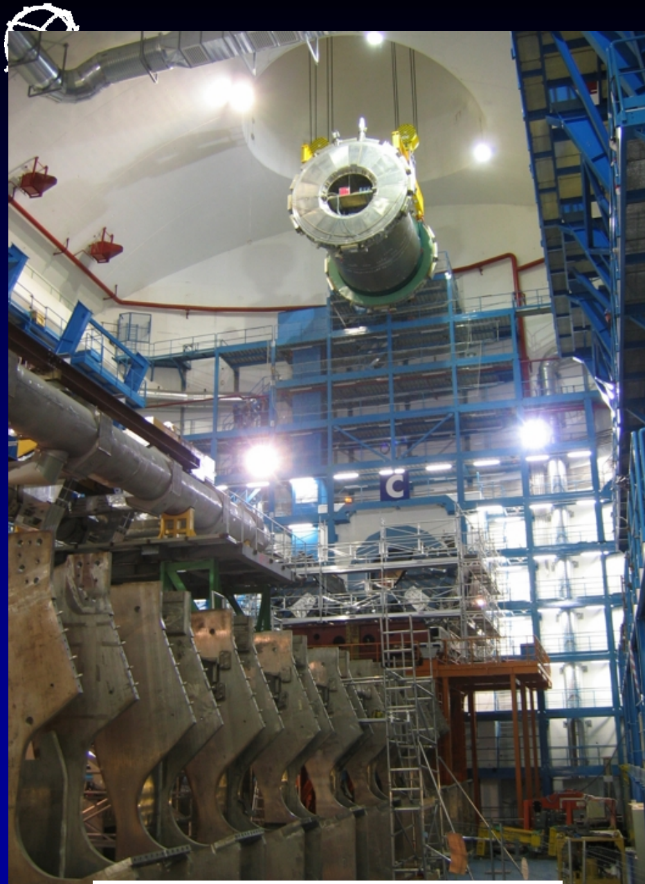
Lowering EM barrel into the pit: October 2004
