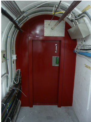
Survey galleries doors and walls
