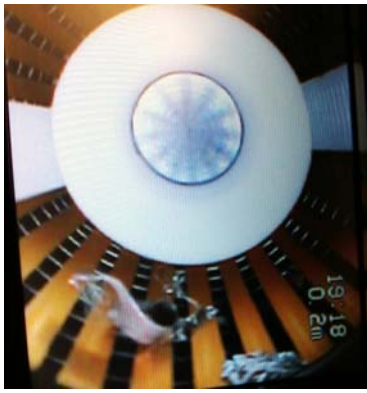
Figure 4: Nozzle blocked by metallic debris
