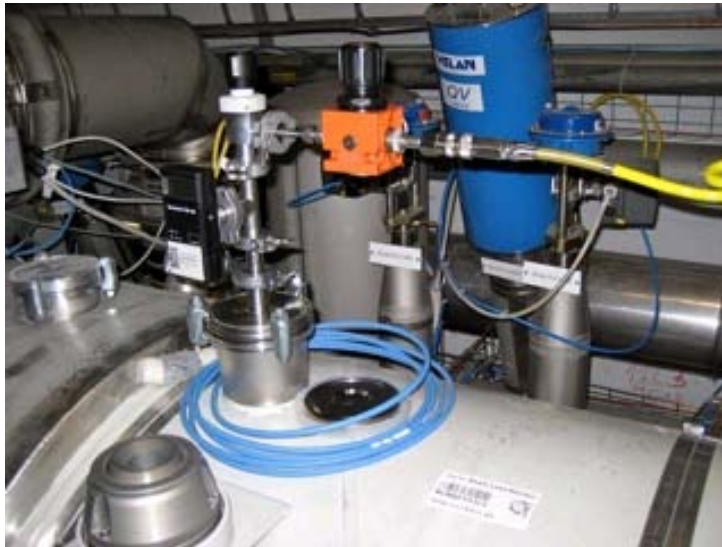
Dry air feed from distribution line
