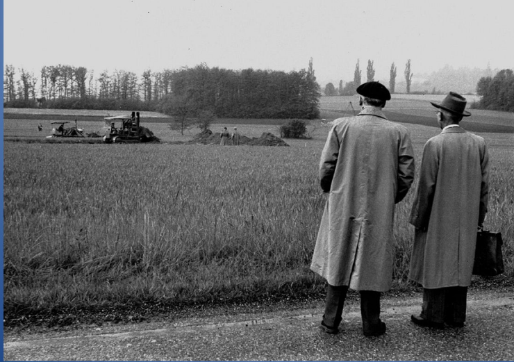
Meyrin Site, start of the works, May 1954
