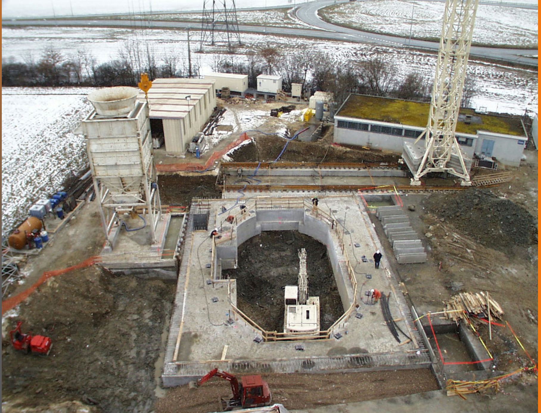
TI2 Area - Start of excavation of PMI 2 shaft - February 17, 1999 - CERN ST-CE
