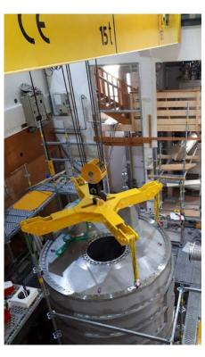
In house trial assembly without thermal shields nor the superconducting coil for leak tests
