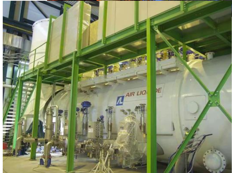
LHC refrigerators: 140 kW @ 4.5 K
