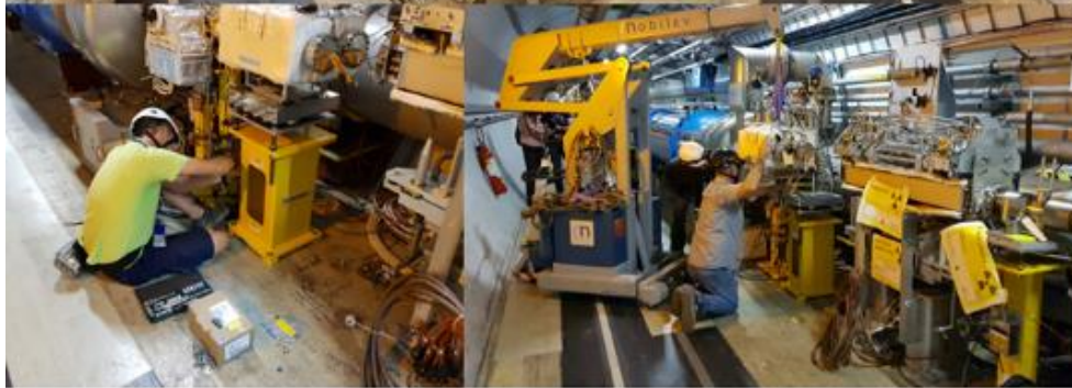
New TANB installed in LHC-IR8
