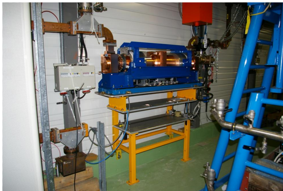
RF power phase shifter in the CLEX gallery
