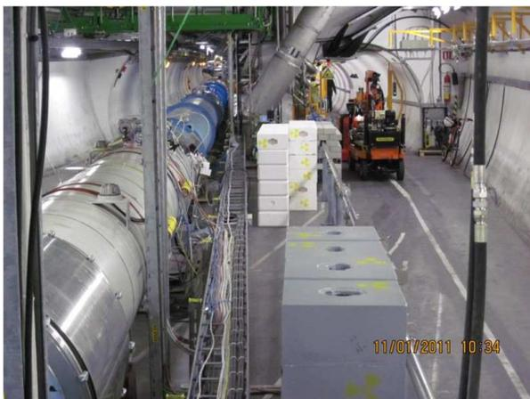
Figure 7: Shielding blocks installed in UJ22. On the right the incoming TI 2 line, upstream view.
